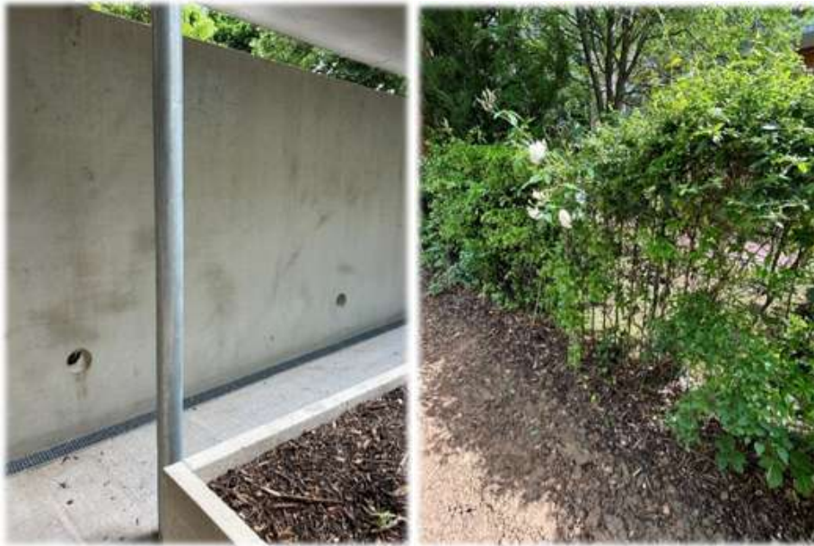
Fence with catwalks (left) and coarse-mesh fence (right): collective housing project, MONTREUIL (93)
