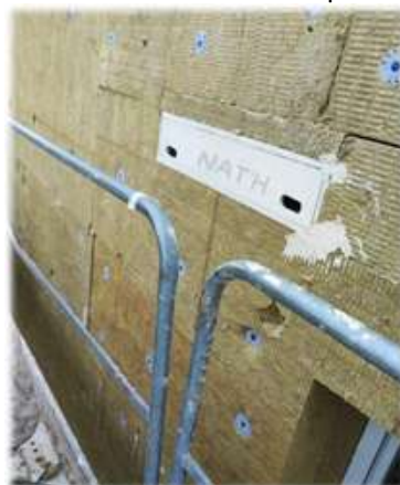
Example of a wooden concrete nesting box for swifts in the ETI
